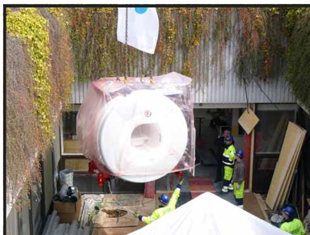
The magnet of one of the new MR scanners being lowered into the hospital building in March 2010.
